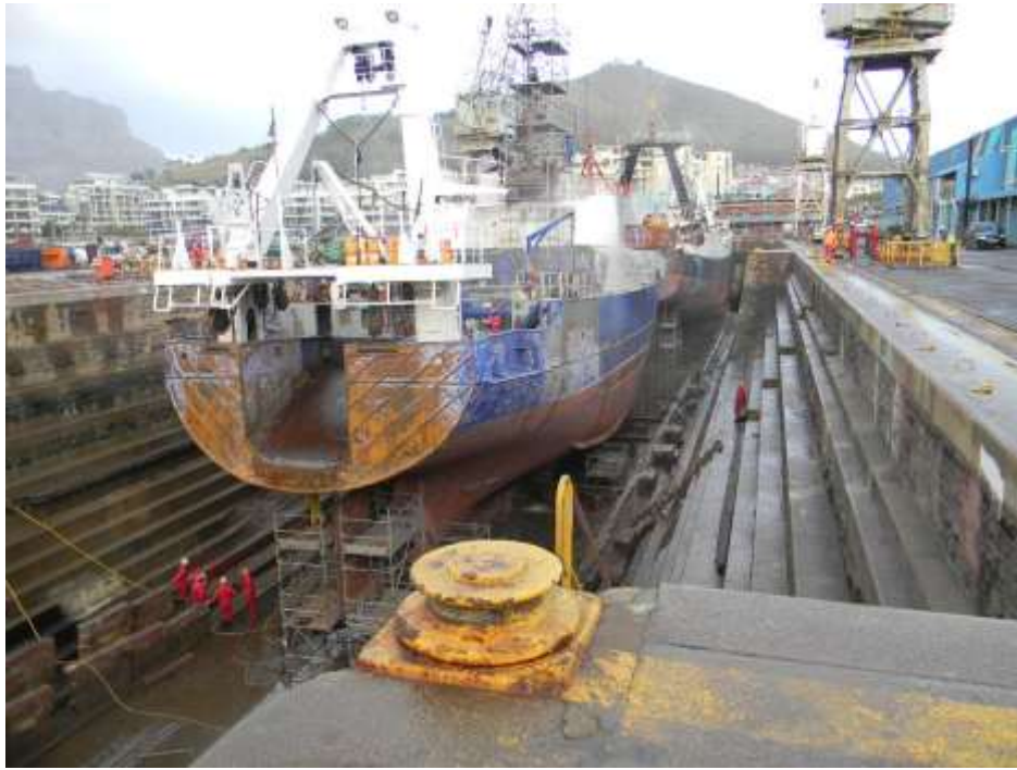
Figure 20: Ship repair in Robinson dry dock, Port of Cape Town (image from [8])
