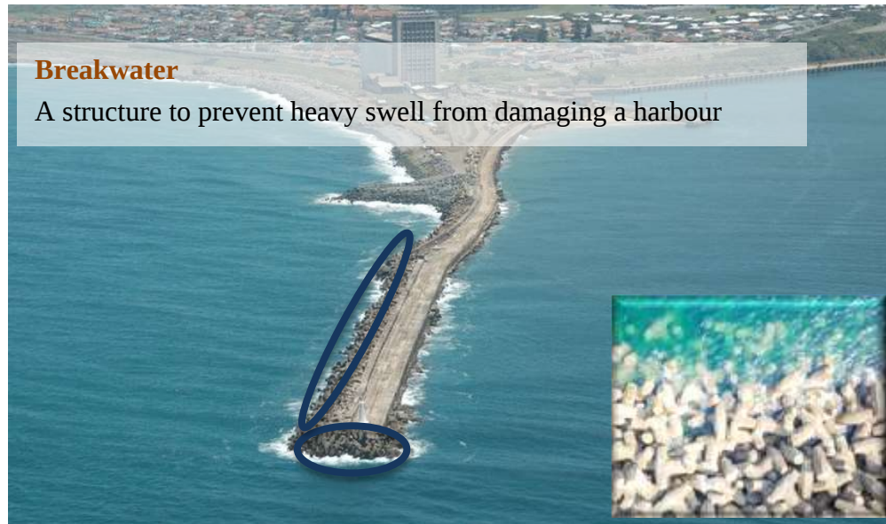
Figure 8: Dolosse breakwater protecting port entrance in East London.
